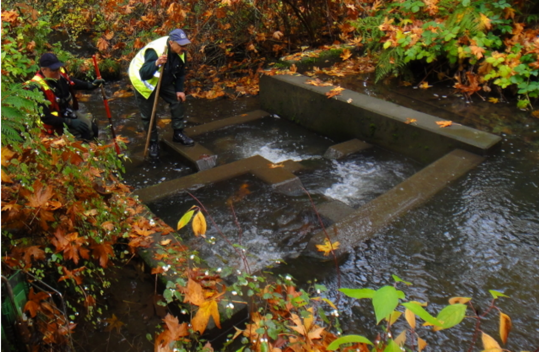
Fish Ladder in Cat Stream
