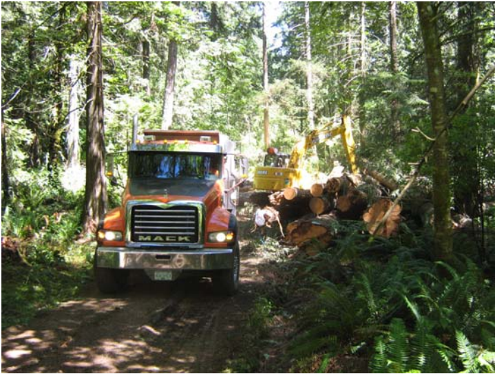
Trucks were used intermittently to haul materials.
