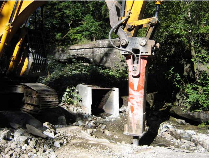
The old fishway was modified and the new channel was connected to the Millstone River at the base of Deadman Falls.
