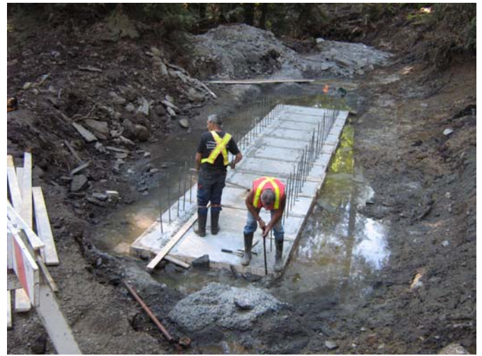
The diversion structure footing was poured first, followed by the walls.
